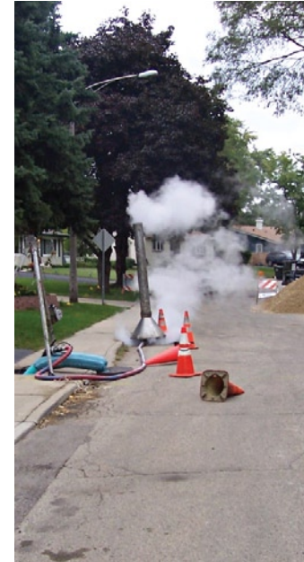
▲ CIPP lining being steam cured
