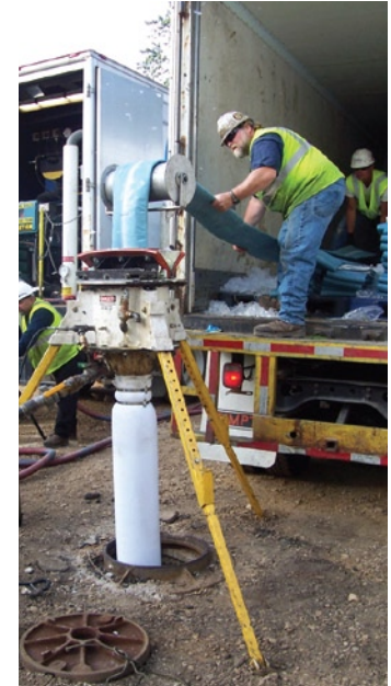
▲ CIPP lining installed in sewer pipe
