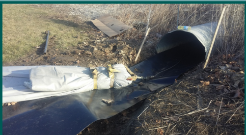
CIPP Liner Folded Over and Getting Ready to be Pulled Through Culvert
