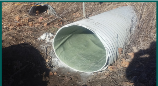
After: Culvert Lined and Liner Cured
