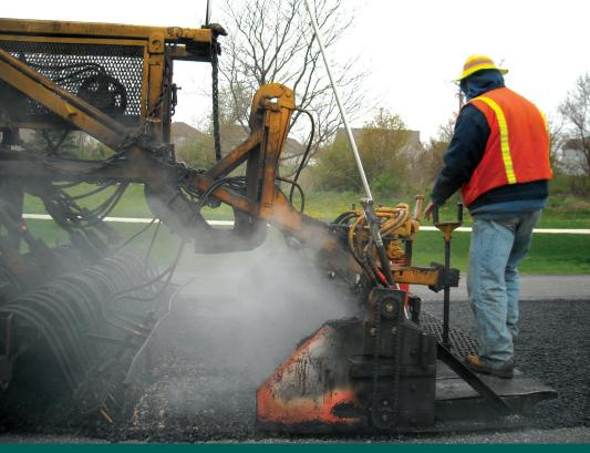
Scarifying unit loosens the heated material
