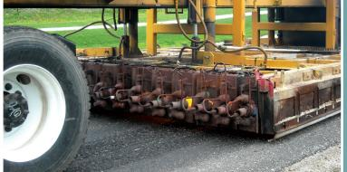
Heating unit heats the existing pavement
