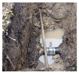
Upon issuance of the IEPA loan, construction commenced on November 7, 2019. New one-inch services were installed via minimally invasive horizontal directional drilling. Copper services were installed from the main to the new curb stop for all houses. From the curb stop to the meter inside the homes, the service was either HDPE with tracer wire (slab foundation; 87 total) or copper (basements; 19 total). New meters were installed and grounded appropriately.
