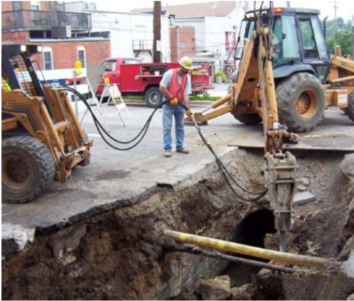
Removal of existing poured-in-place concrete
