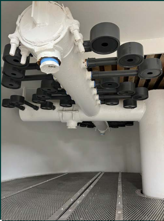
Fully recoated aerator with new nozzles and spray trays
