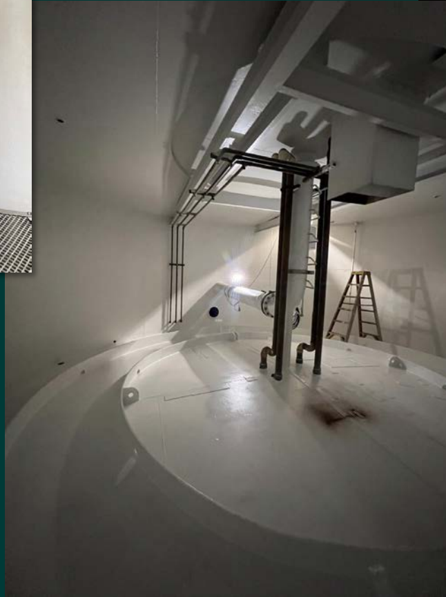
Fully recoated exterior and all new valves and actuators
