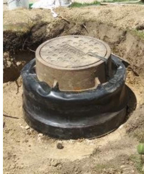
External Chimney Seal
