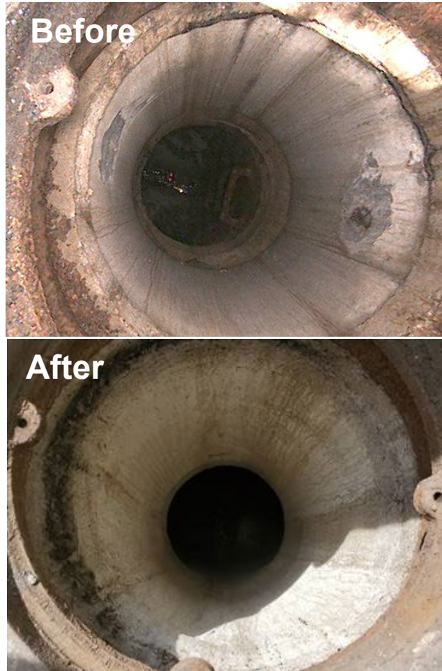
Manhole Rehabilitation
