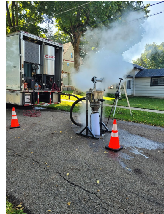
Sanitary Sewer Main Rehabilitation
