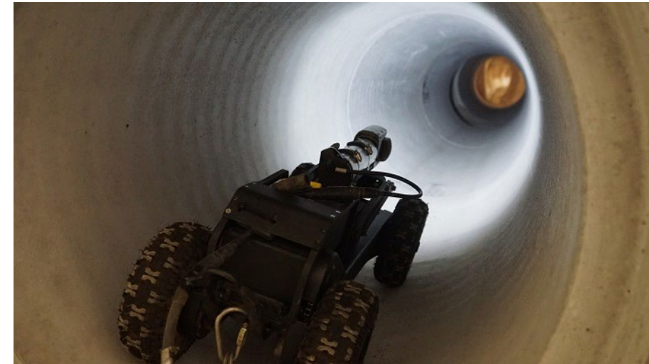
Sanitary Sewer Main Televising
